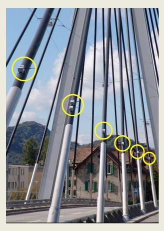
Structural monitoring is increasingly applied on civil structures to provide reliable and quantitative data about their actual performance. This data is used in the assessment, maintenance and rehabilitation efforts of bridges that are approaching the end of their design lifespan. Conventional wired monitoring systems turned out to be inflexible, labor-intensive and expensive.
